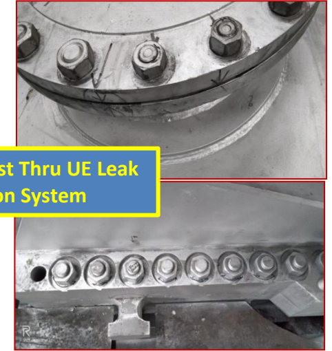
Air Ingress Points in TG Circuits
