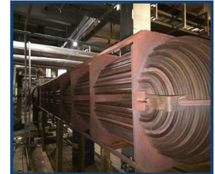
HPH-5 Internal Inspection
