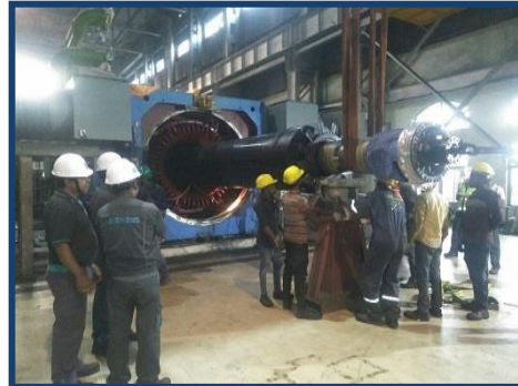
Rotor Thread out
