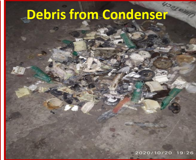
Post Condenser Cleaning
